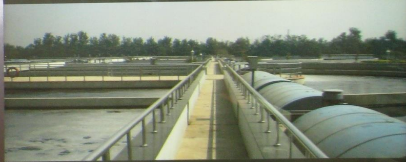
China • Langfang Wastewater Treatment & Water Recycling Plant Capacity: 80,000m 3 /day (wastewater treatment), 40,000m 3 /day (water recycling). Completed: 2007
